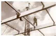
Stressed concrete beams, rather than steel, were used in the structure. The containing walls are brick and he chose rustic flettons as they weather well, and he strengthened these walls with buttresses containing a concrete
